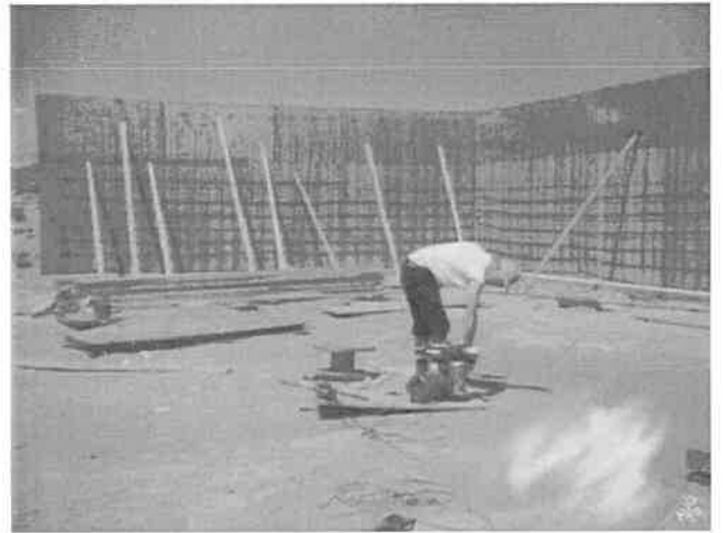
Forming the North and West walls of the building 1979.
