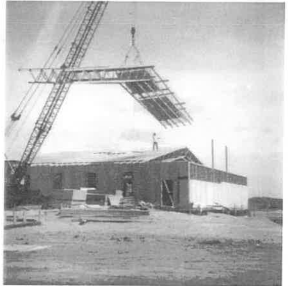
Crane lifts final roof section into place. Done August, 1980.
