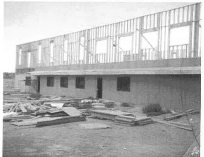
Building takes on second floor.
