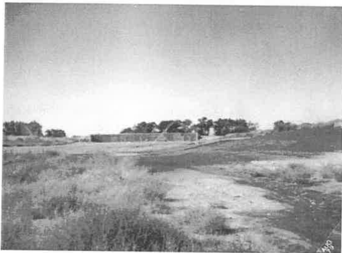
Looking north over the future ball field to the north wall form of the building.
