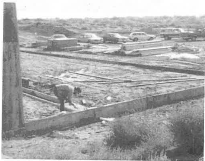
South wall footings and wall forms.
