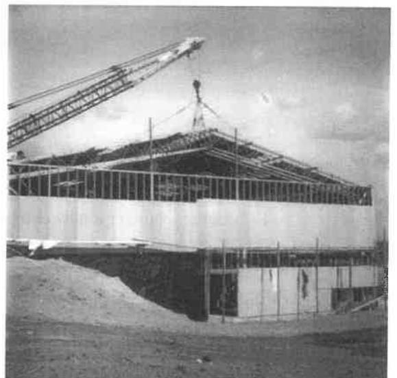
Final roof section in place.
