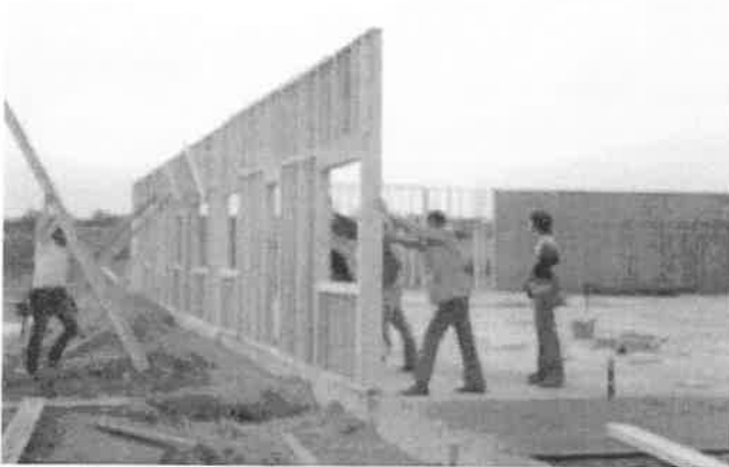
Framing the South side.
