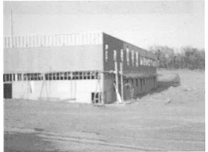
Second floor gets framed. Looking from the northeast. Taken spring 1980.
