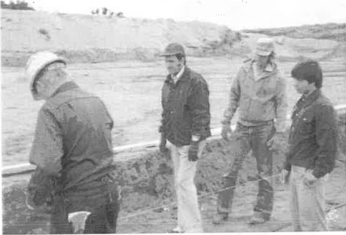
Tom Roberts, Bob Lovett, Johnnie Lovett and helper lay out footings.
