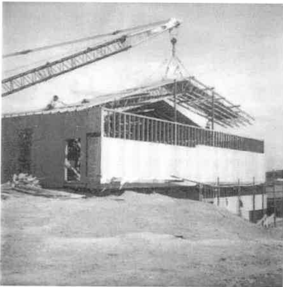
Another view of crane placing final roof section into place.
